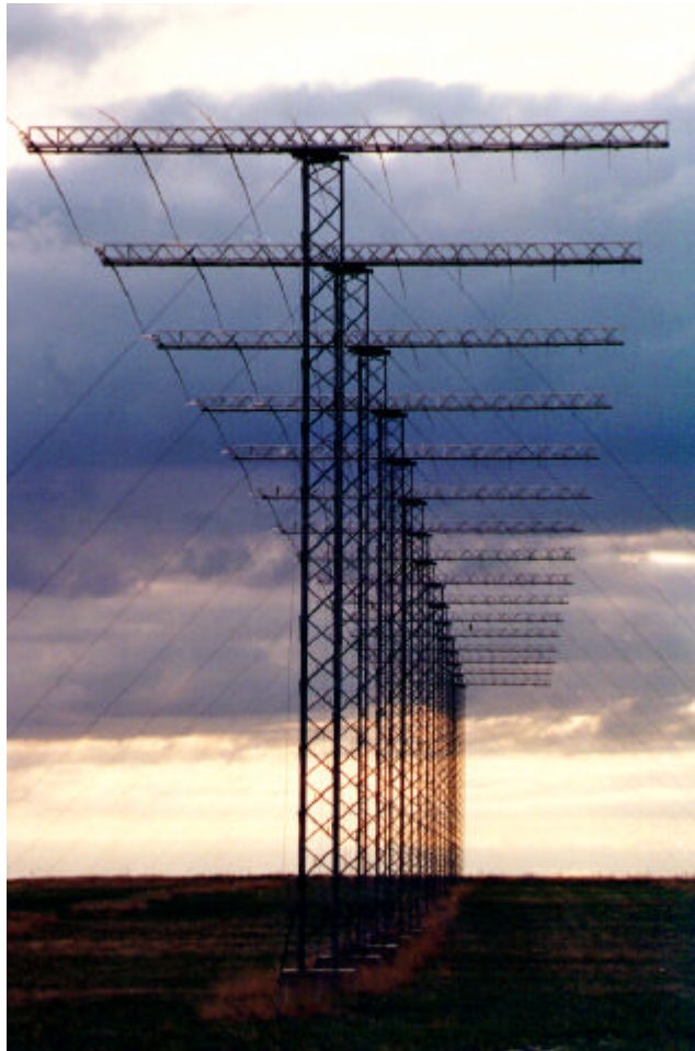
Figure 5. Antenna of the Saskatoon SuperDARN HF radar collect signals from the space environment and help scientists understand the energy circulation driving space weather.
